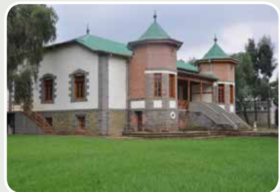
Renovation of the EAs Headquarters
