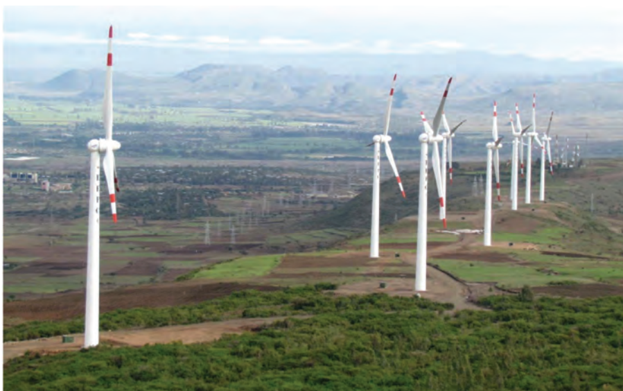
Figure 2.4: Adama I 51 MW Wind Farm (34 WTGs each generating 1.5MW)
